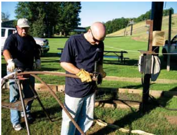
Cutting rope with grinder.
